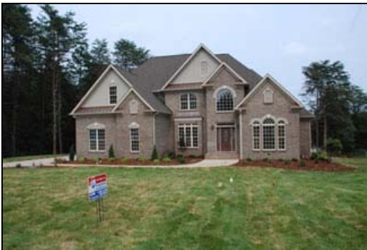
Exterior landscaping is now complete
